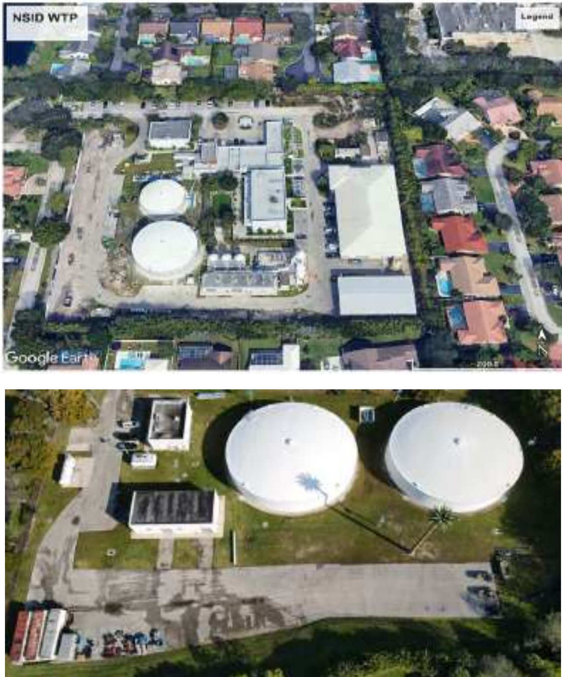
Figure 3.4 — Water Treatment Plant and Booster Pumping Station Aerial Views
